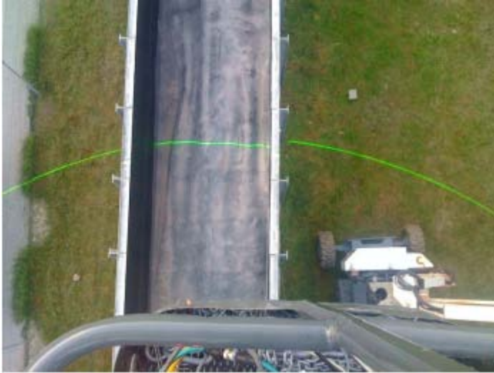
Figure 5: View from the cabin of the boom lift down to the empty basin. The scan line of the laser scanner is visible on the ground.
