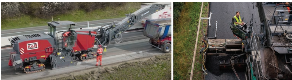
Abb. 6: links: 3D-Asphaltfräse, rechts: 3D-Asphaltfertiger.
