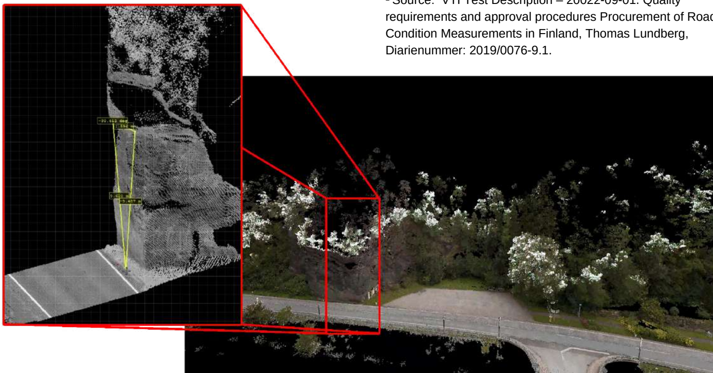
Figure 6: RIEGL Mobile Mapping point cloud data: High resolution coverage of the road infrastructure as well as the surrounding terrain. The zoomed area shows a rock formation close to the clearance profile of the road.
